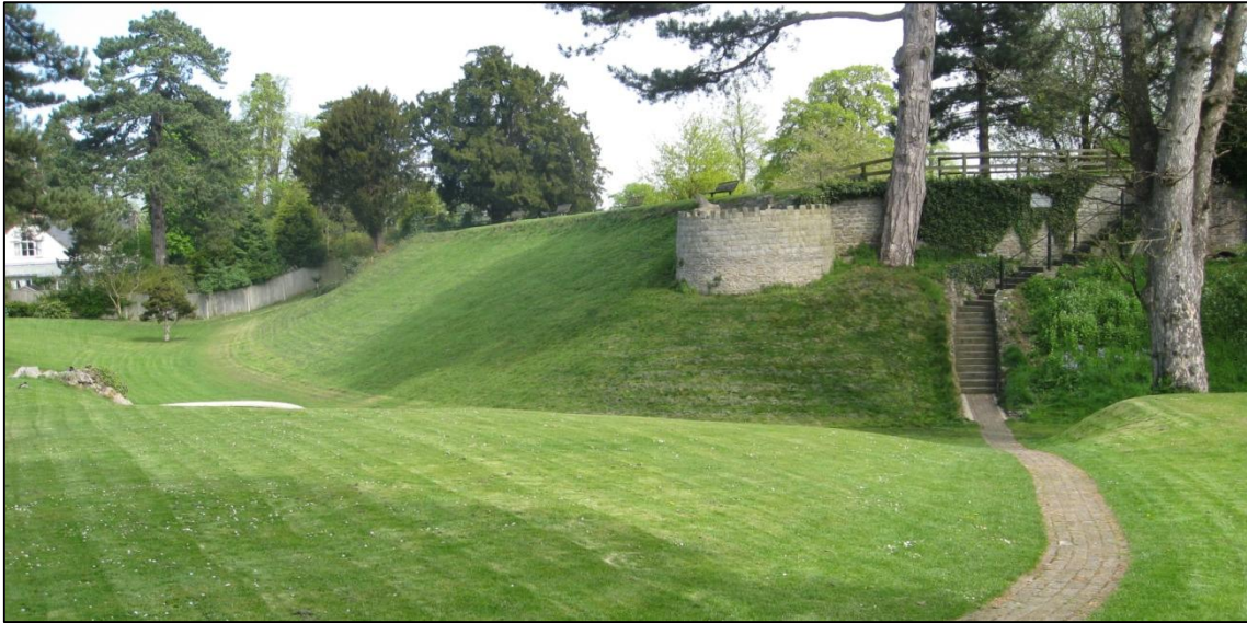
Figure 4.11 The ramparts of the south-western bailey from the south. When first constructed in the twelfth century the bailey area and its ramparts were significantly lower, and were only raised another c.1-2m in height in the thirteenth century. In the left-hand side of the image the gable end of The Coach House can be seen; fragments of walls possibly associated with the thirteenth-century castle were identified encased within the walls of this late post-medieval building (Source: Michael Fradley).
