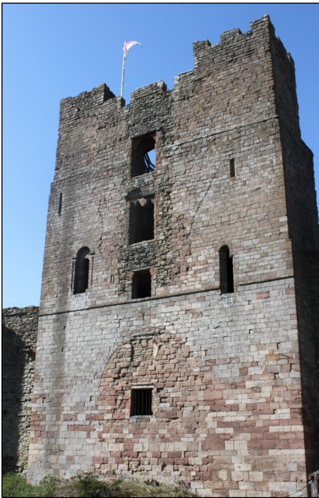
Figure 4.10 The twelfth-century tower gate at Ludlow Castle, Shropshire. The infilled archway of the large original gate can be seen at the base of the structure (Source: Michael Fradley).
